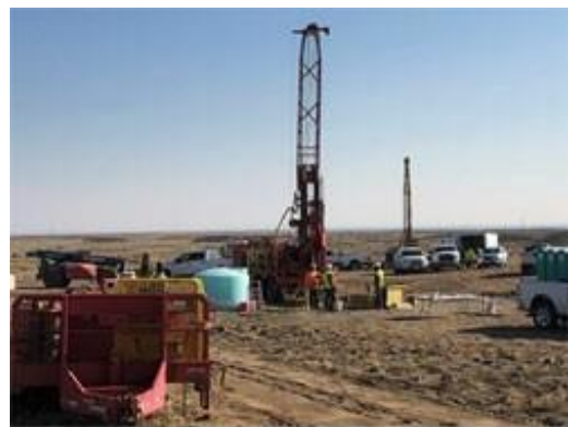
Core boring drill rig
